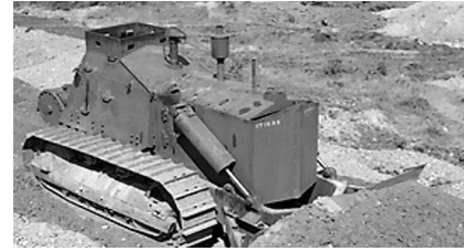
D-7 Armored Bulldozer
